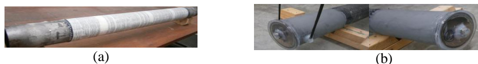
Figure 3. (a) Curing with masking tape for 24 hours, (b) Sealing of ends to prevent corrosion inside
