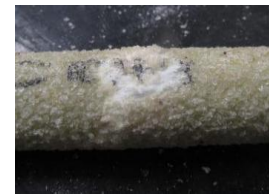
Figure 8. Crushing of the resin and fibres of GFRP bars (100 °C to 150 °C)
